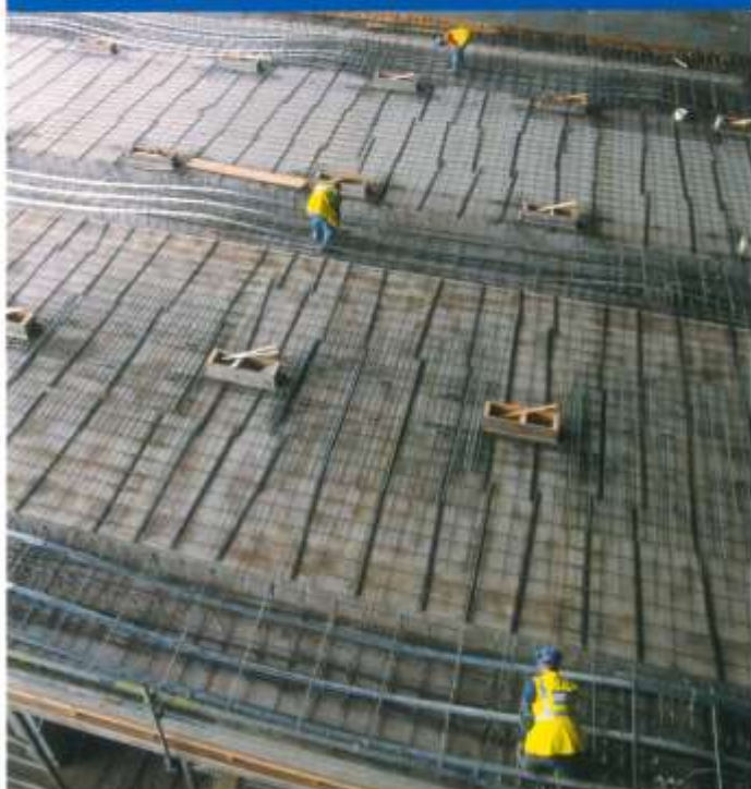
Installing prestressing cables
