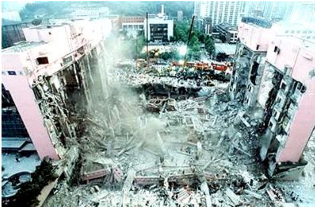
Figure 4 The Sampoong Department Store collapse [12]
