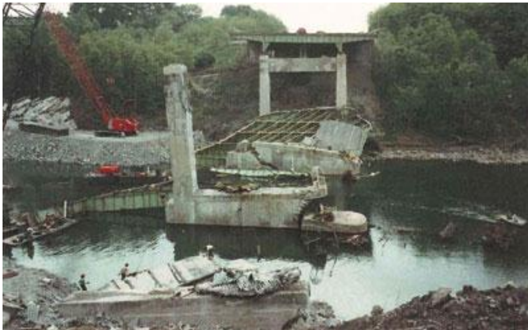
Figure 3 Schoharie Creek Bridge collapse [12]
