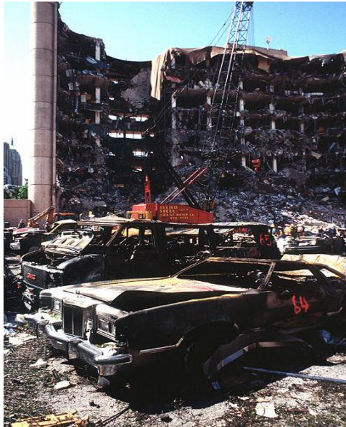
Figure 5 Alfred Murrah Federal Building collapse [12]
