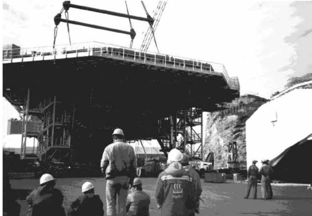
Helideck, Helihangar, Stairtowers and Support Structure
