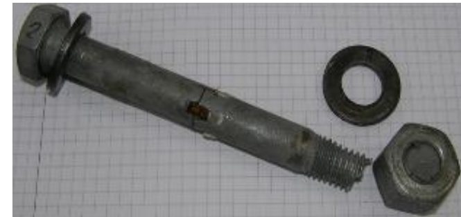
Rupture of bolt close to nut
