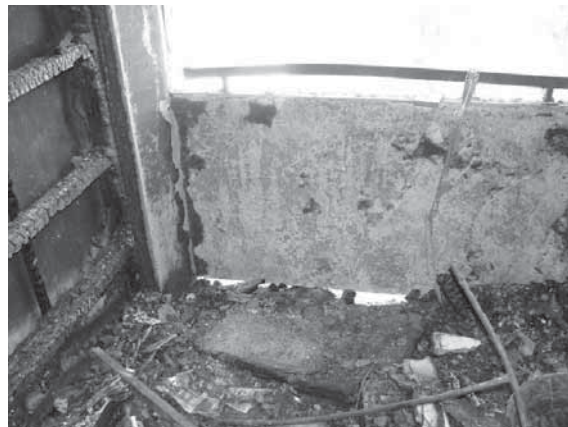
Fig. 11.10 Irregular additional insulation on the side wall of the loggia
