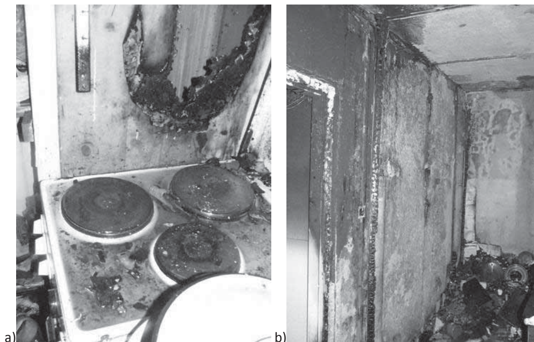
Fig. 11.3 a) The kitchen was the starting point of fire, b) The kitchen on the next upper storey after the fire case
