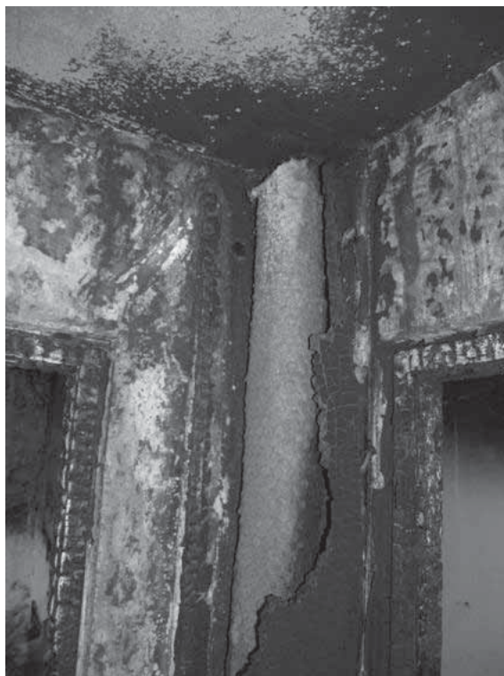
Fig. 11.15 Floor penetration without seal after fire
