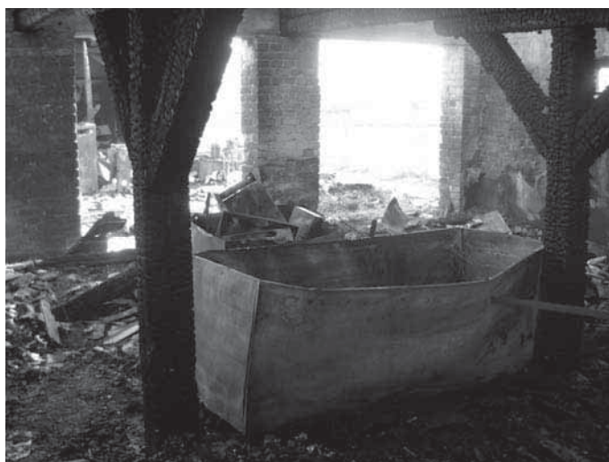
Fig. 4.2 Burnt refrigeration appliances and the roof structure
