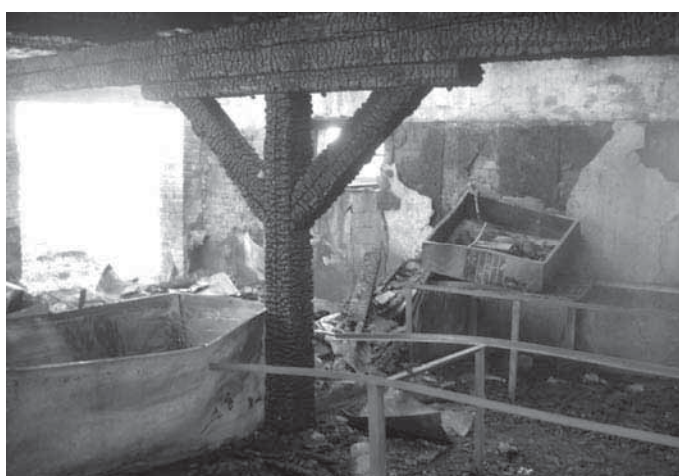
Fig. 4.1 Burnt refrigeration appliances and the roof structure
