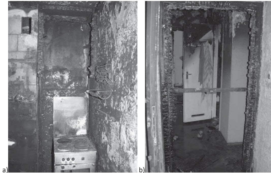
Fig. 11.7 a) The kitchen and b) the entrance door after the fire
