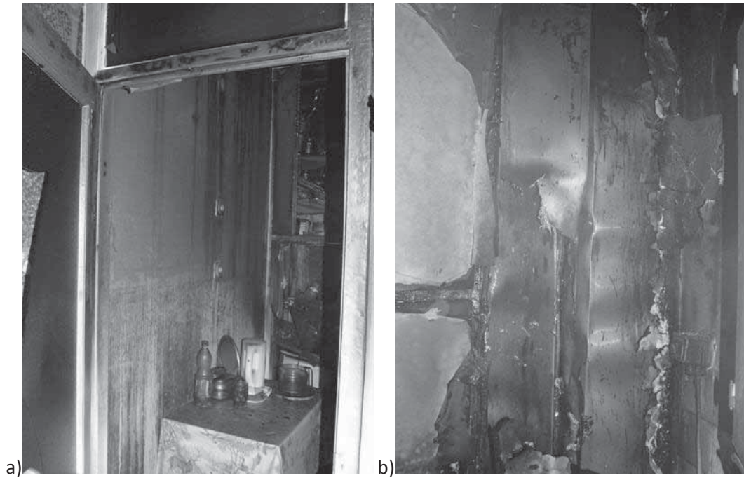
Fig. 11.5 a) The V. floor kitchen and b) the shared air-shaft of kitchen and bathroom looking from the V. floor's kitchen after the fire
