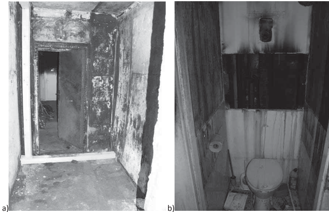
Fig. 11.9 a) Starting point of the fire b) the toilet after fire
