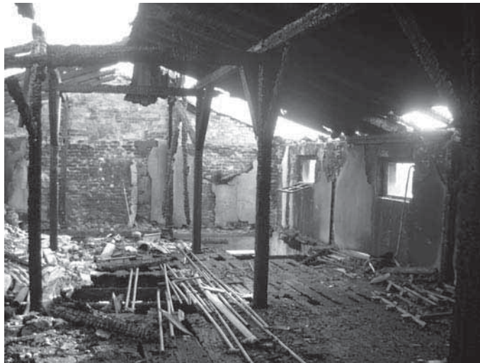
Fig. 4.4 Burned floor and roof structure of the attic
