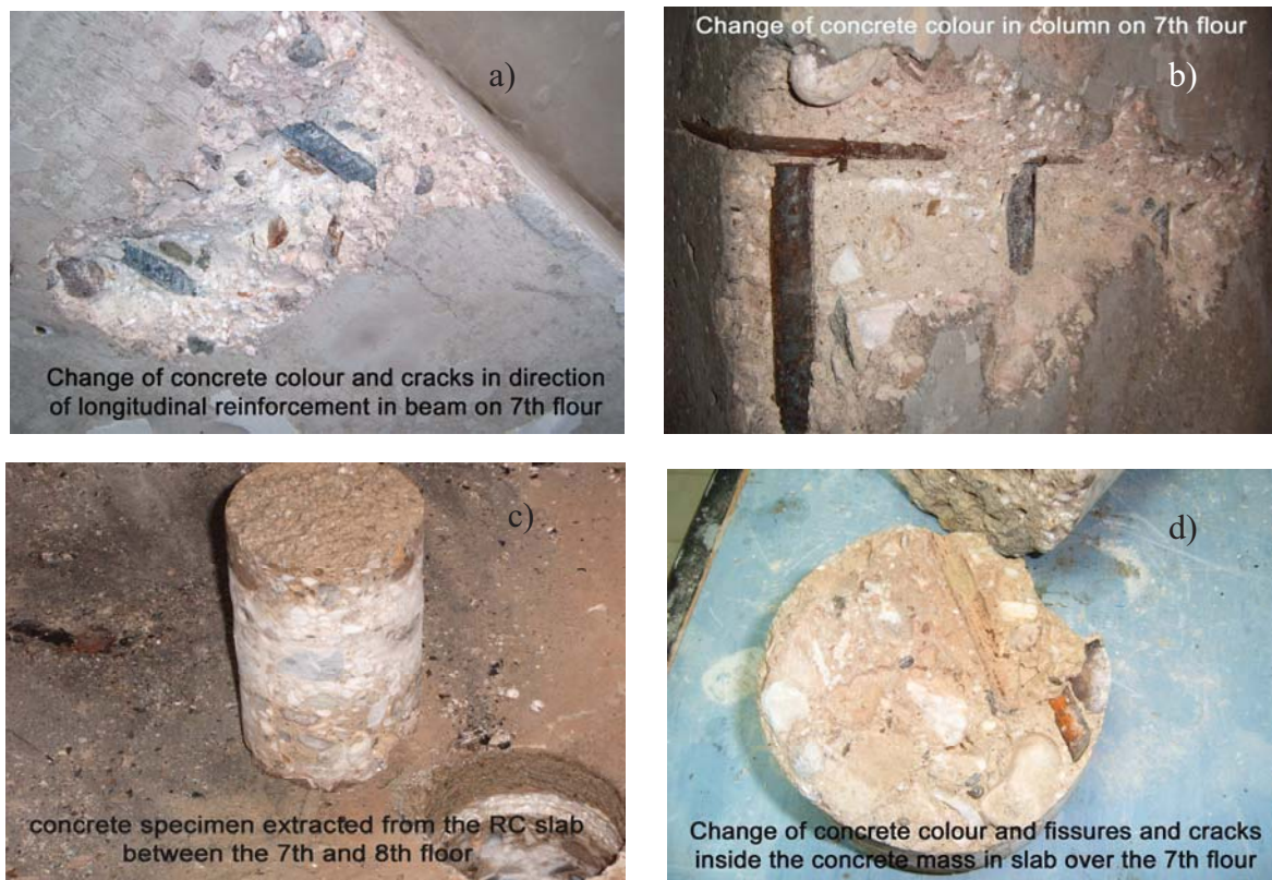
Fig. 31.1 Change of concrete color and characteristic damages of RC elements, recorded in situ
