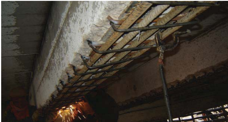
Fig. 30.16 Additional stirrups of beam B2, welded for the existing one.
