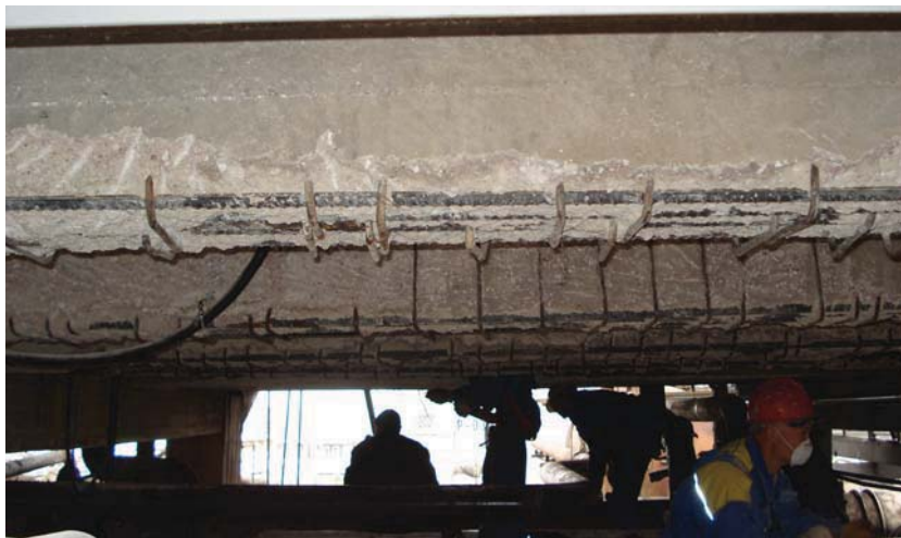
Fig. 30.13 Elimination of the deteriorated (burned) concrete layers up to the main reinforcement
