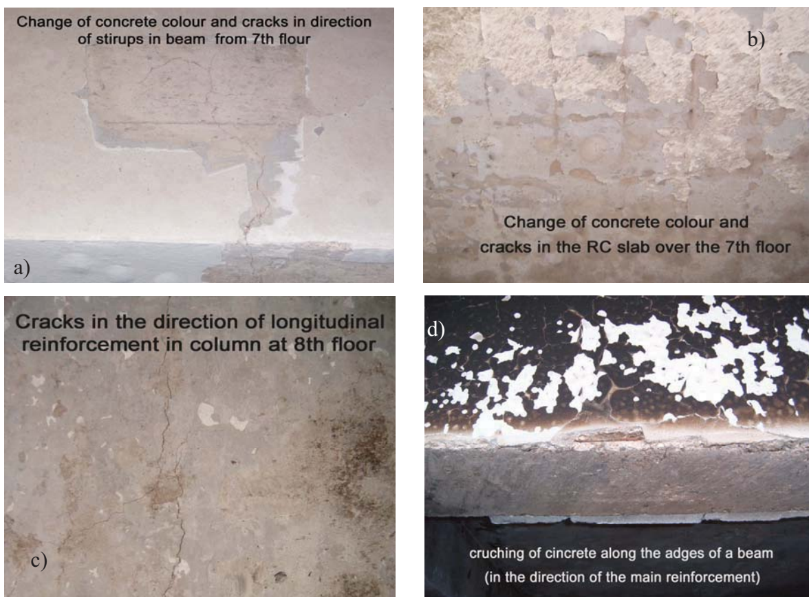
Fig. 31.2 Cracks along main reinforcement in columns, beams and slabs, recorded in situ
