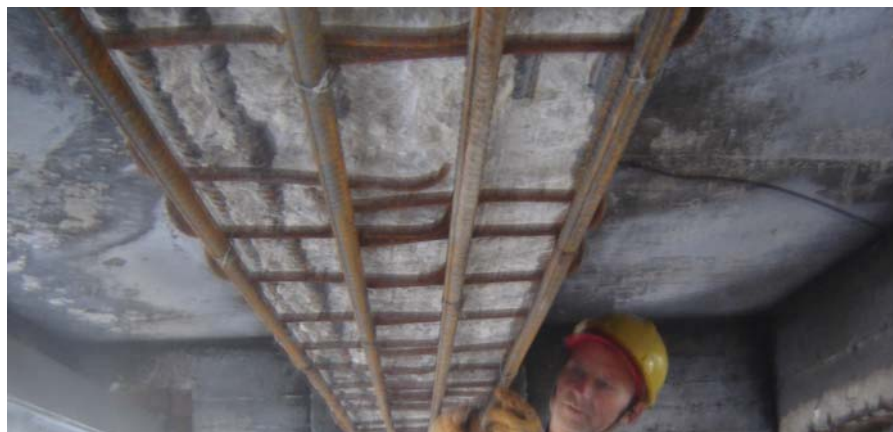
Fig. 30.14 Repair of the beam B2 at the second spam.
