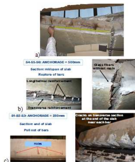
Figure 10: Slab S5 viewed from furnace after test. slab anchorage (a) 500mm; (b) 250mm.
