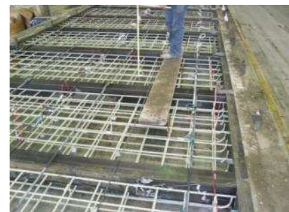
Figure 8: Slabs reinforcement grids before casting.
