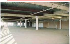
40 to 55% of beams can be left unprotected by placing protection where it is needed.
