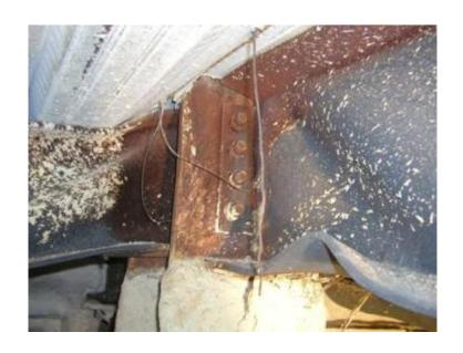
Lower flange buckling occurred during early stages of fire – thermal expansion
