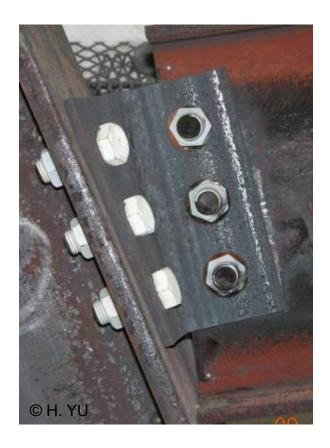
Double web cleat for unprotected beams
