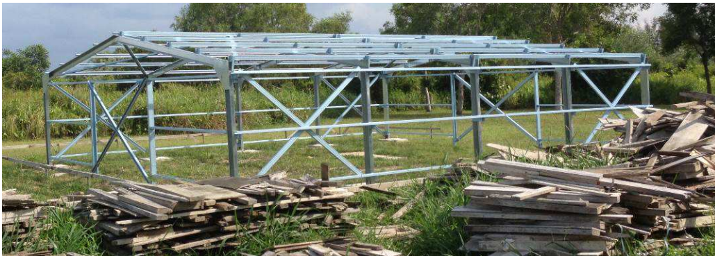
Fig. 4 - Full scale site fire test frame
