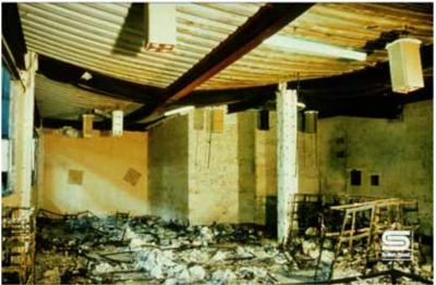
Deformed state of the heated part of the composite floor
