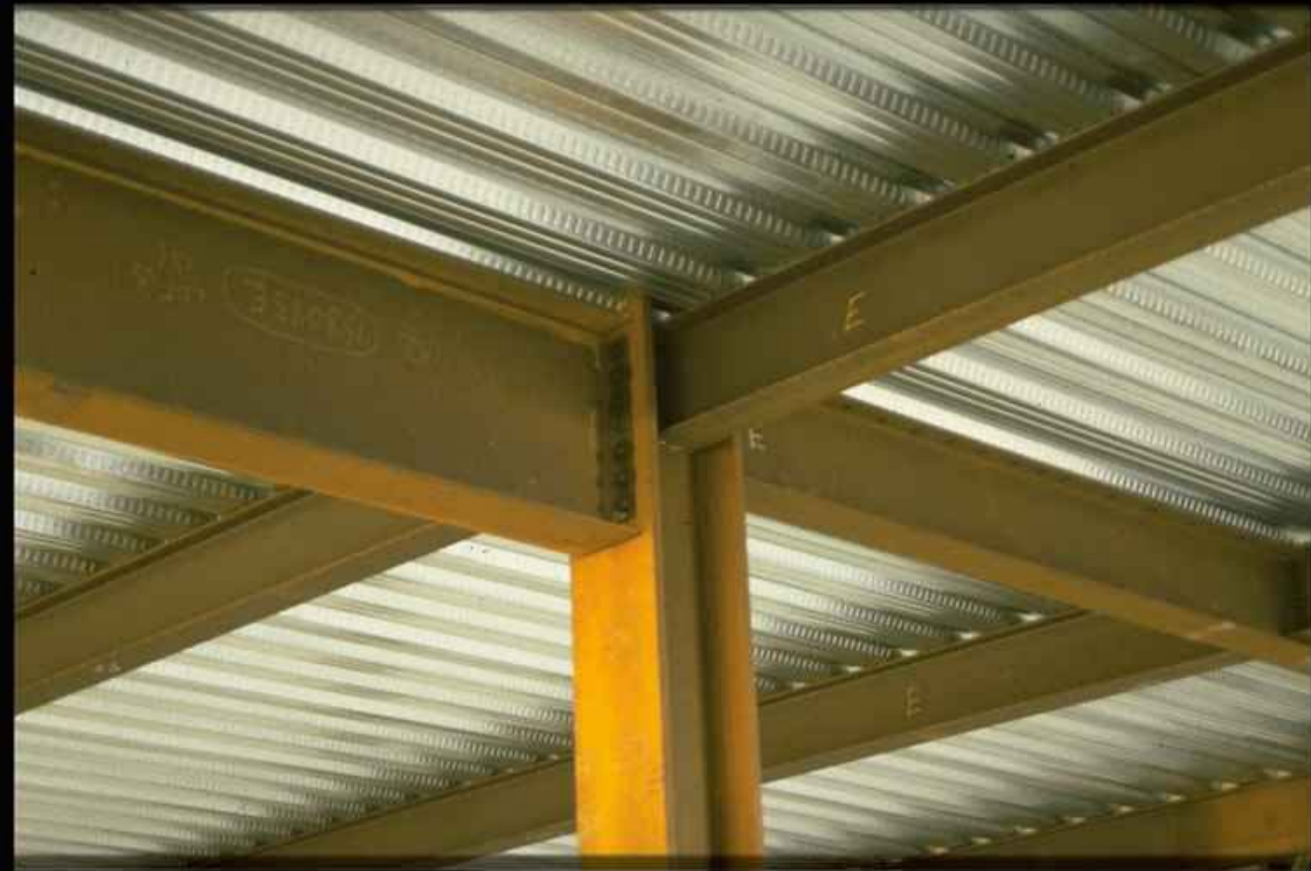
Typical composite structure
