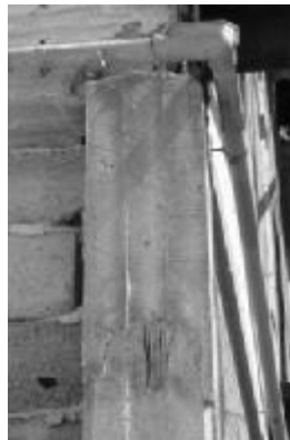
(b) Repaired end column
