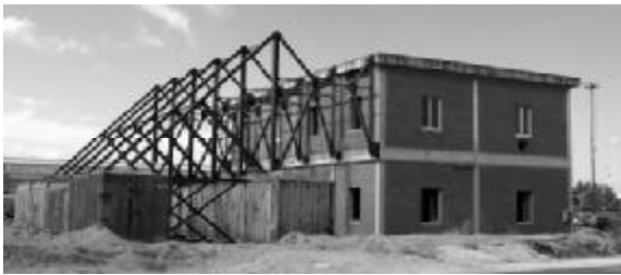
Figure 3. R.c. building for full scale tests in Naples (Italy).
