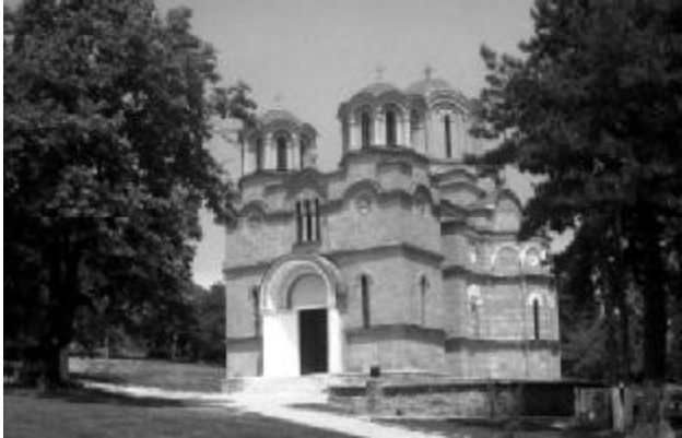
Figure 15. Southwest view of reconstructed church
