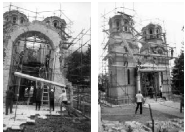
Figure 14. Repair of the belfry towers
