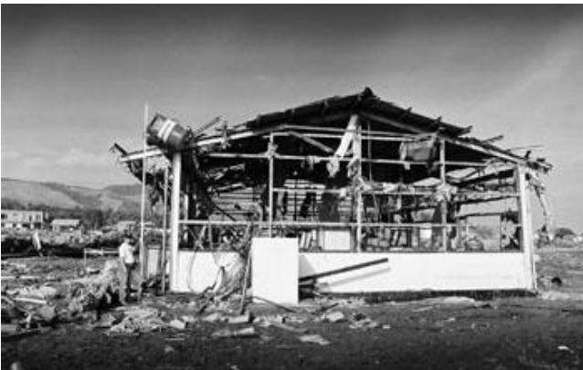
Figure 5. Example of a tsunami effect on a house. Credit: Dr. Jose C. Borrero, USC Tsunami Research Group, courtesy NSF.
