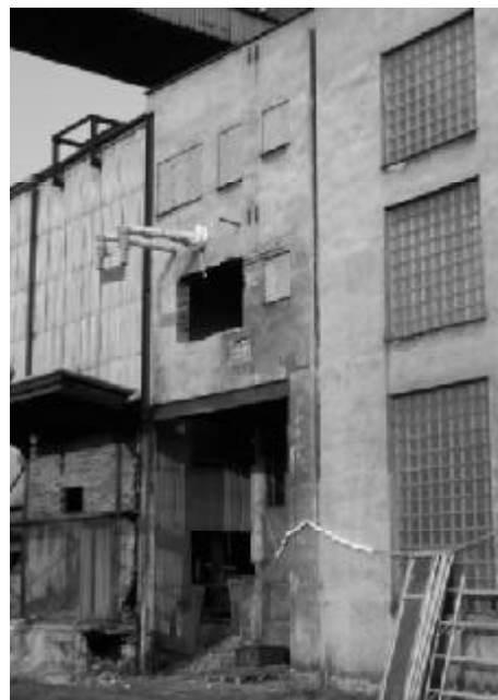
Figure 1. The fire compartment on the 2 nd floor of the building.
