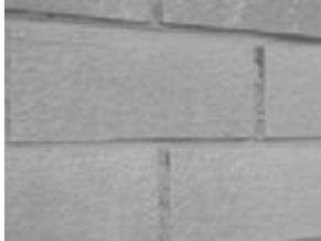
(a) Grinding of joints
