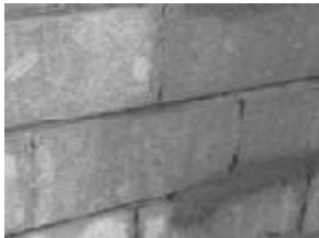
(c) Application of “Emaco® Formula Tixo”
