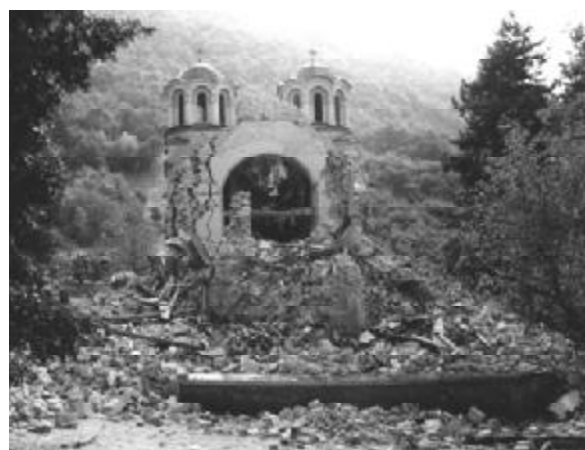
Figure 2. Southeast view of the demolished church
