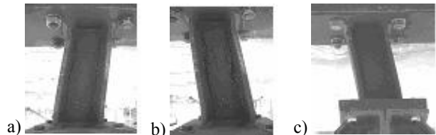
Figure 16. Test No.3 on EBs: damage pattern.
