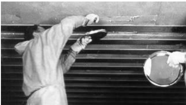
Figure 2.5. Application of CFRP strips on building floors.
