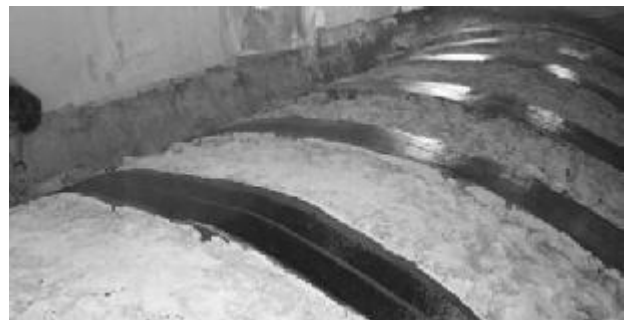
Figure 2.11. Strengthening of a historic vault with CFRP strips.
