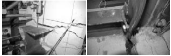
Figure 7. Collapse of the joint (hogging) under biaxial loading
