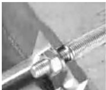
Figure 5. Wire mesh geometry and texture and chemical anchor
