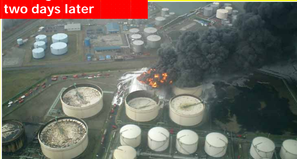
▲ Figure 1. Aerial view of the fire in the oil tank damaged by long-period ground motions from the 2003 Tokachi-oki, Japan, earthquake (courtesy of Dr. Hiroshi Koseki, National Research Institute of Fire and Disaster, Japan).
