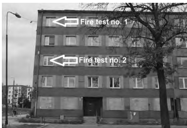
Fig. 1 External view of the building
