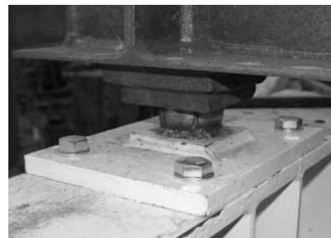
Fig. 4 Fixed pin point support
