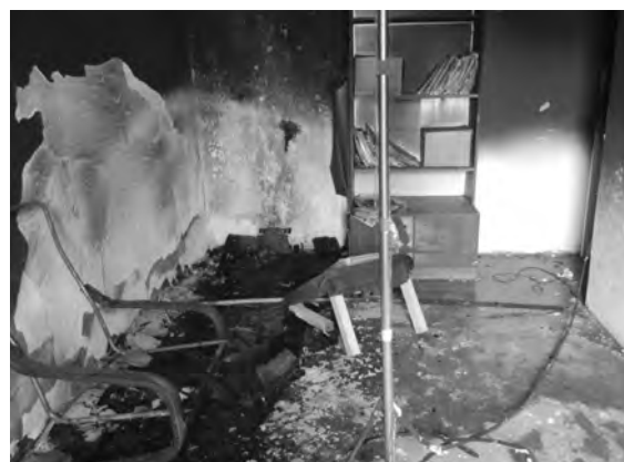
Fig. 6 Fire compartment after test no.2
