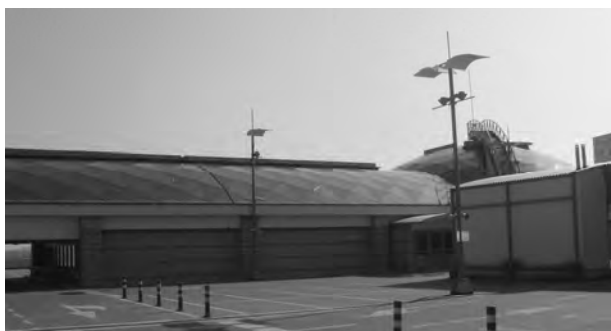
Fig. 1 Braced barrel vault in the Atrium Promenada Shopping Center
