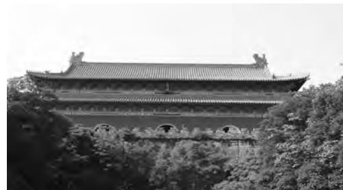
Fig. 2 Rebuilding roof with ancient shape
