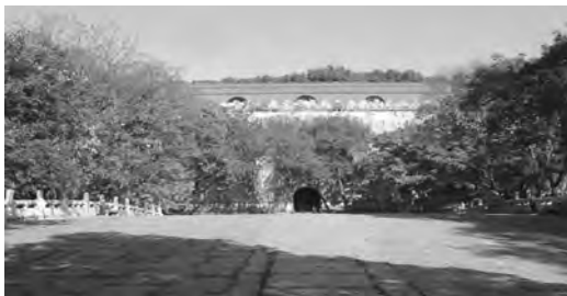
Fig. 1 Minlou building without roof
