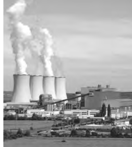
Fig. 2 Tušimice power plant
