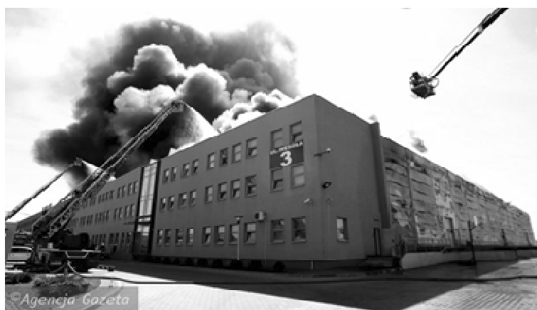
Fig. 1 View of the complex during the firefighting (internet source); in the foreground the administrative-office part of the building is seen
