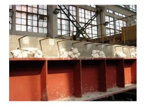
*Fig.4.* Anchorage of the reinforcement at the boundary of the slabs
