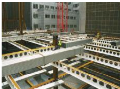
Fig. 1. Use of cellular beams in buildings
