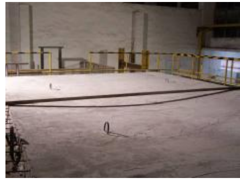
Fig.14. The deformation of the slab after the test
