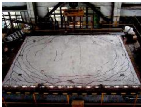
Fig.19. The cracks on S-4 after the test
