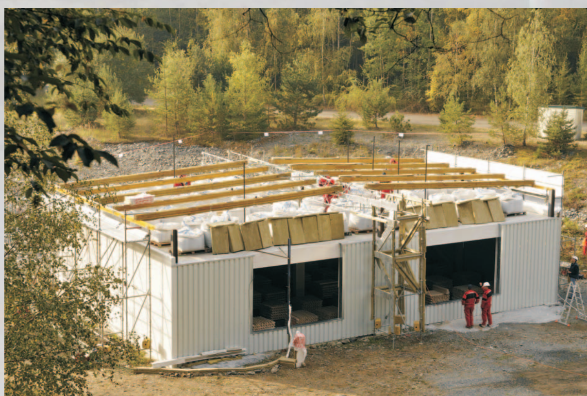
Overall view of the experimental building with scaffolding for measuring deflections
