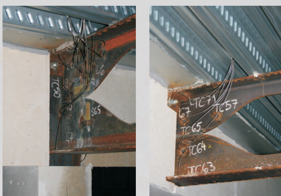
Beam to column (A) and beam to beam (B) connections with thermocouples
