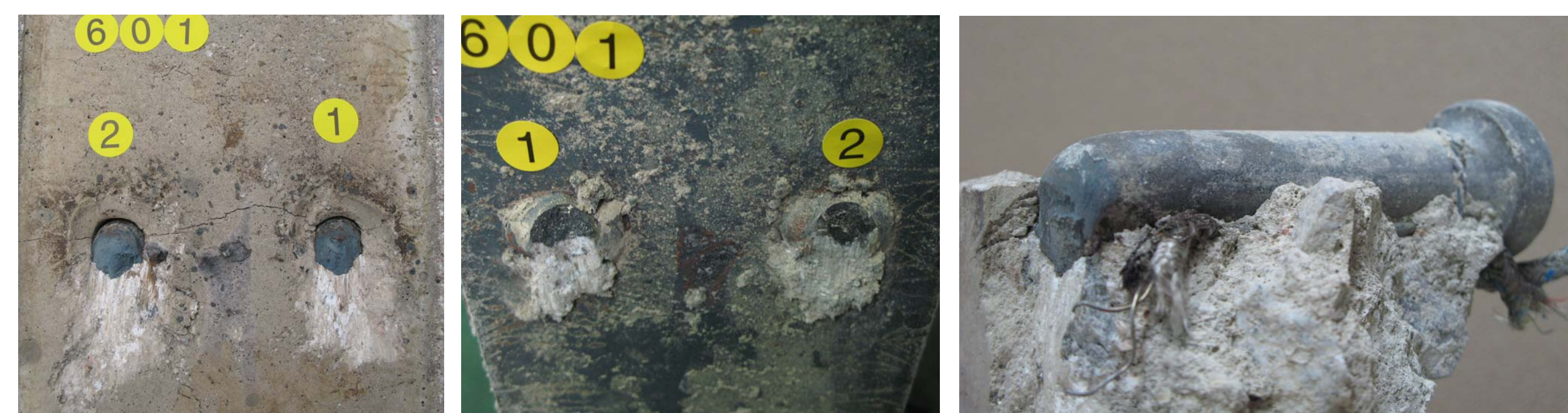
Fig. 6. Failure of stud shear connector after push-out test at 60 minutes of the standard fire
