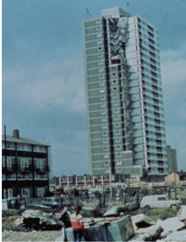
Figure 1. Progressive collapse - Ronan Point.
