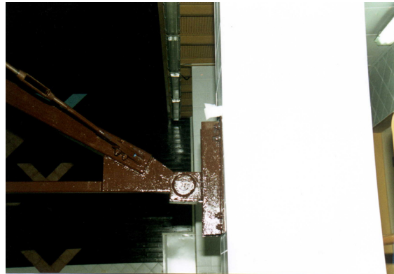
Fig.5 The hinge of supporting truss
