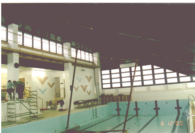
Fig.3 Temporary supports of purlins
