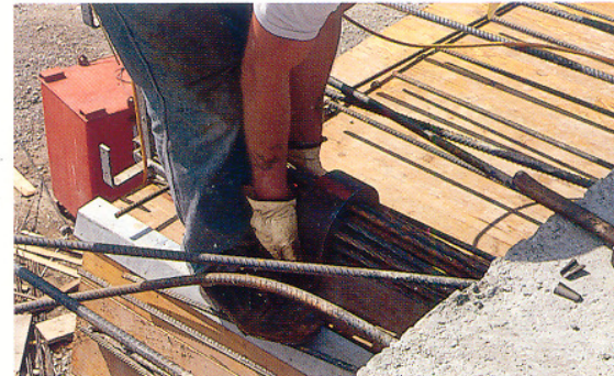
Placing of anchor head
