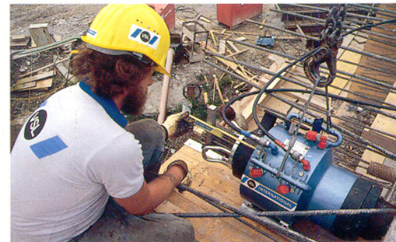
Stressing, measuring, seating of wedges
