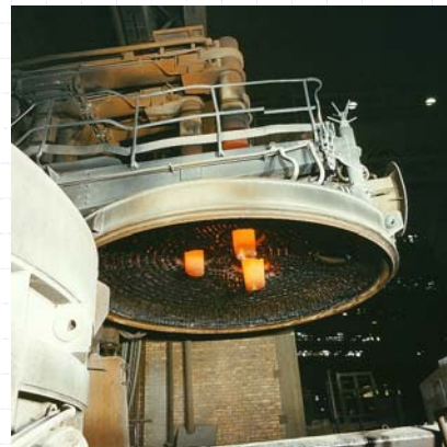
The roof of an arc furnace removed, showing the three carbon electrodes
