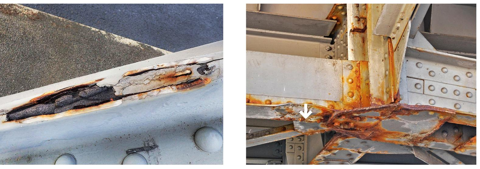
Diagonal deformation due to crevice corrosion
