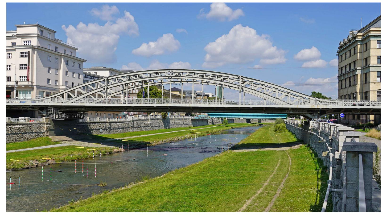
On the remains of the pylons, a simple arch truss structure was anchored with a length of 59 m and a bridge deck width of 5.5 m. Damage repair, the design of the new structure, its manufacture and installation were carried out in a surprisingly short time. The riveted steel bridge spanning the River Ostravice was completed within four months and came into service on the 8th of January 1887. It was designed and built by the bridge factory of Vítkovice Ironworks.
