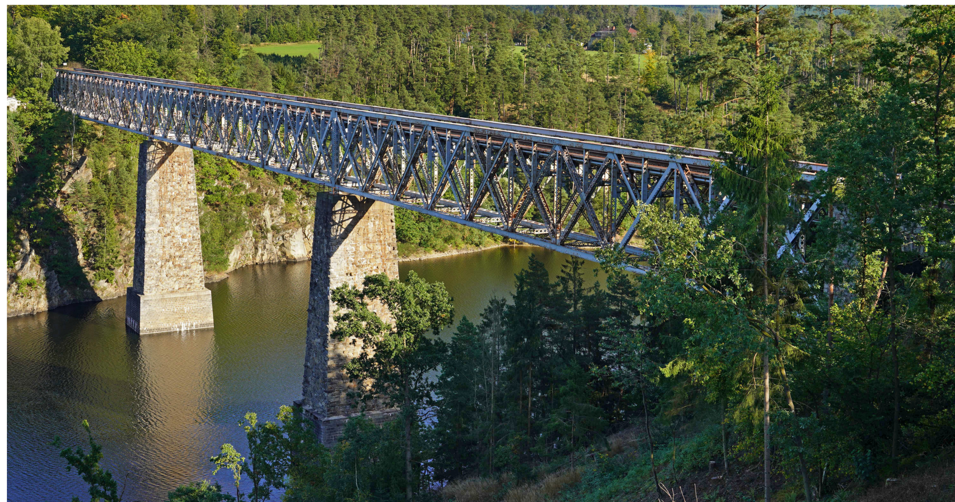
View of the bridge from the northwest
