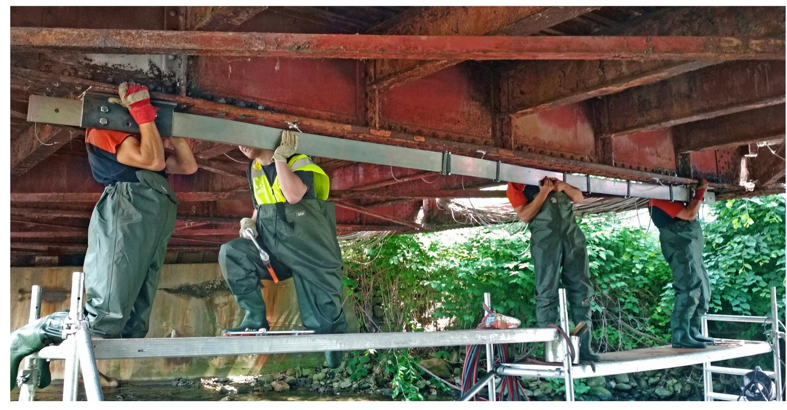
Strengthening crossbeam of historic steel bridge with Shape Memory Alloys
