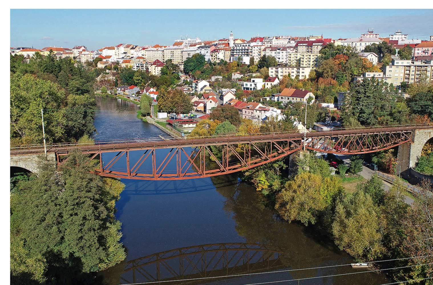
Truss bridge in Tábor (1903) The first electrified railroad track in Central Europe
