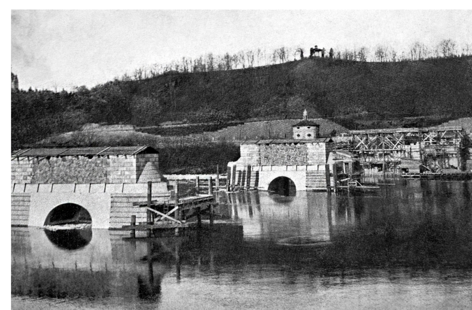
Construction of Čechův most in Prague (1907-1908)
