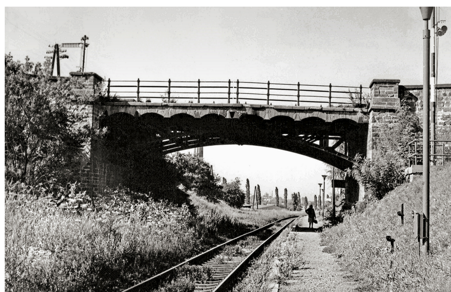
Cast iron bridge near Nemilany and Hoštěhrádky-Řešov
