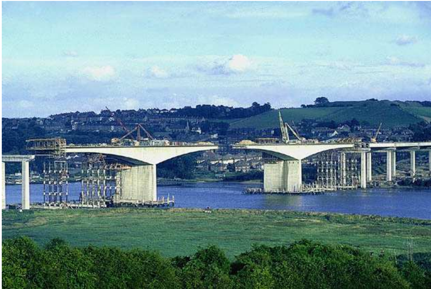
Cantilevered construction of the bridge
