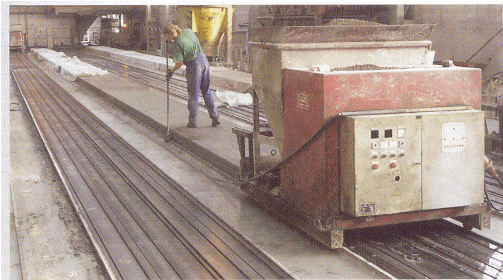
Casting of SPIROLL hollow-core slabs.
