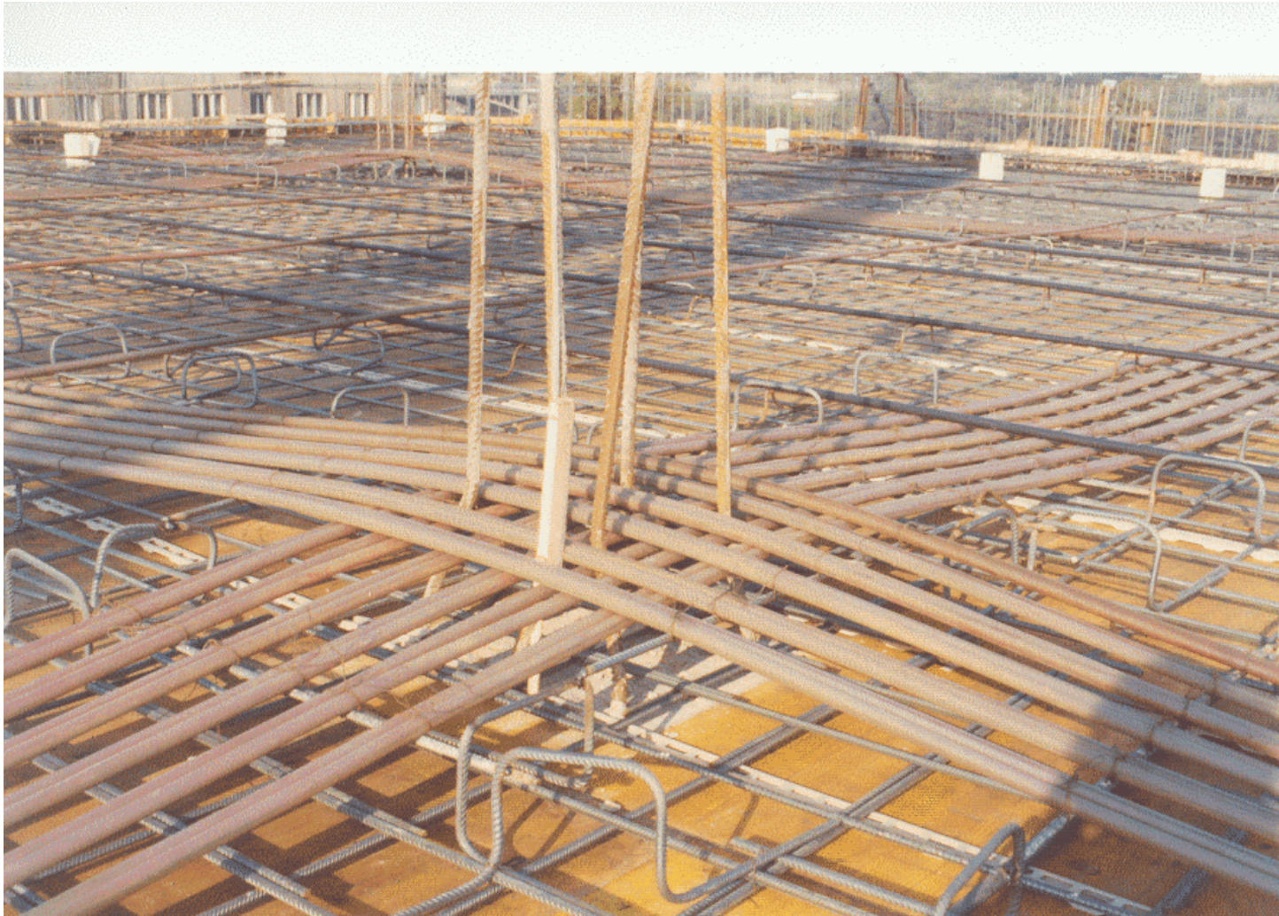
Lift-up tendons over the support
