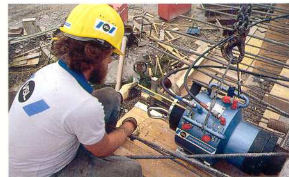
Stressing, measuring, seating of wedges
