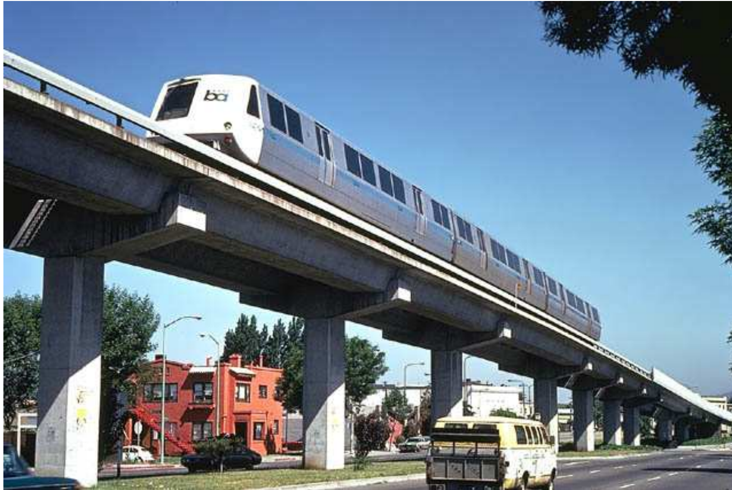
Bridge from the composite postensioned beams
