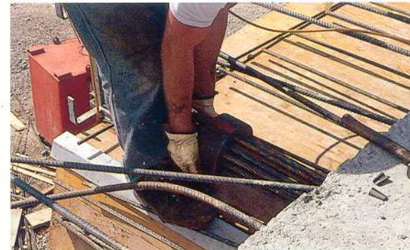
Placing of anchor head
