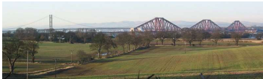
Firth of Forth Bridge (1890) 206+47+518+ 82+206 [m]
