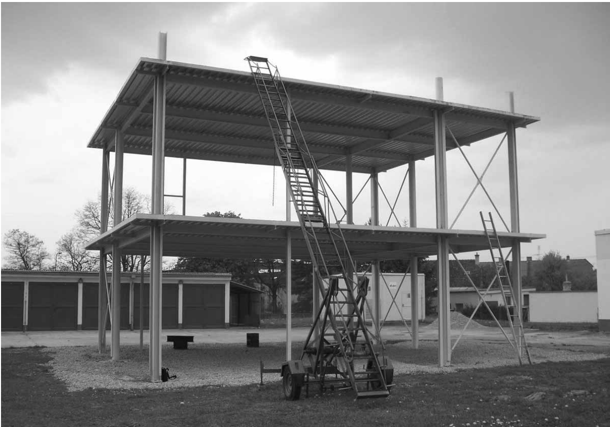
Fig. 28 The steel structure with the composite slabs
