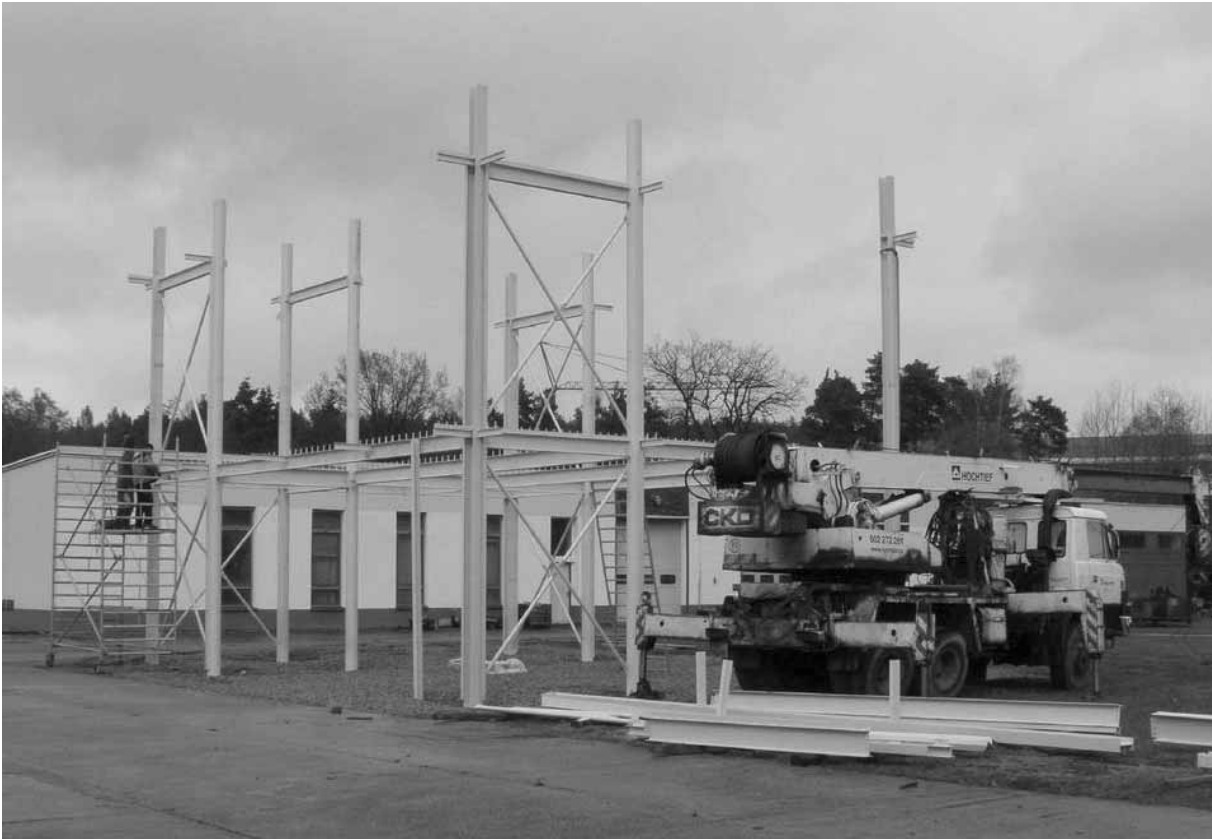
Fig. 25 Erection of the steel structure
