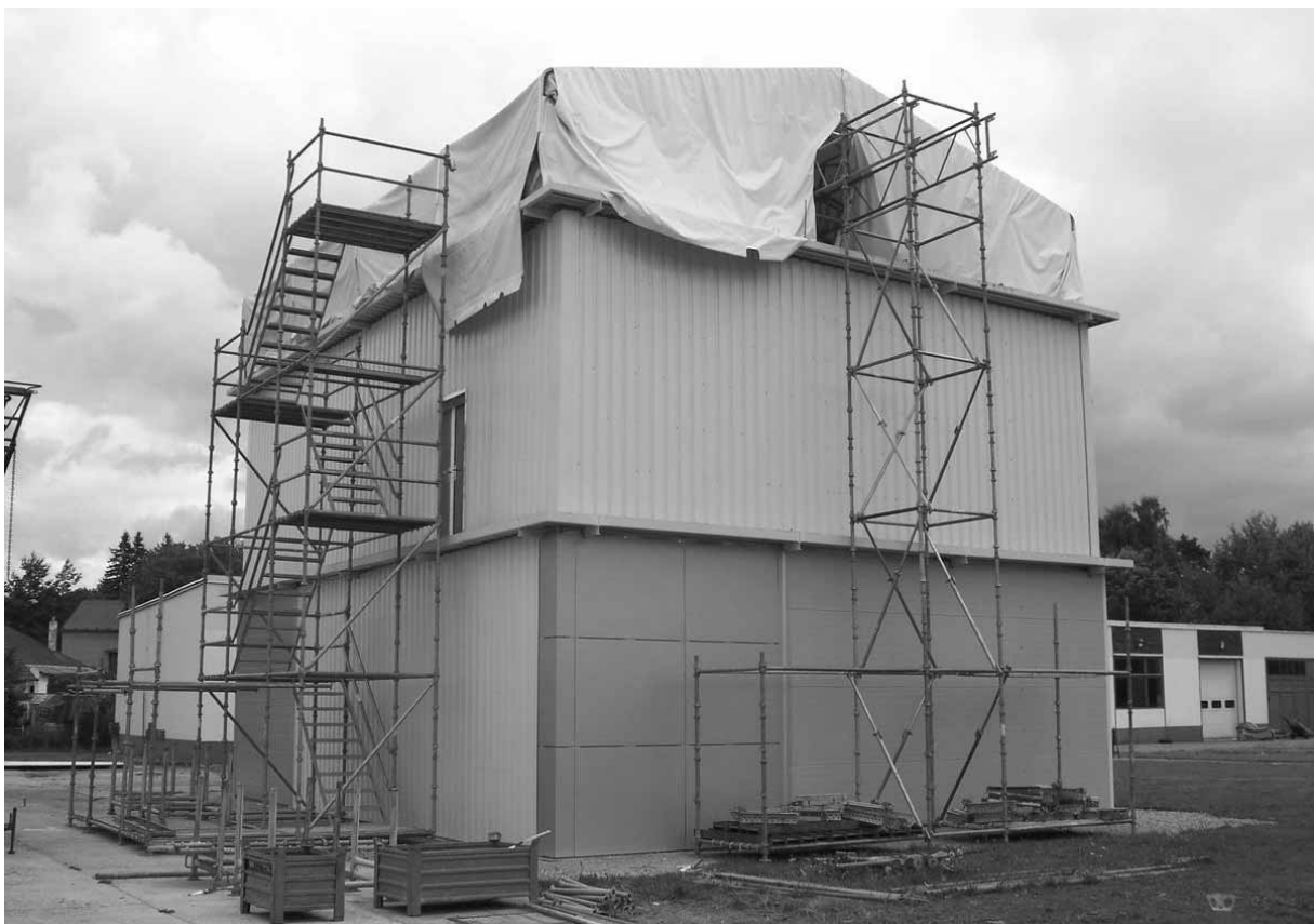
Fig. 32 Frame for measurements and stair tower
