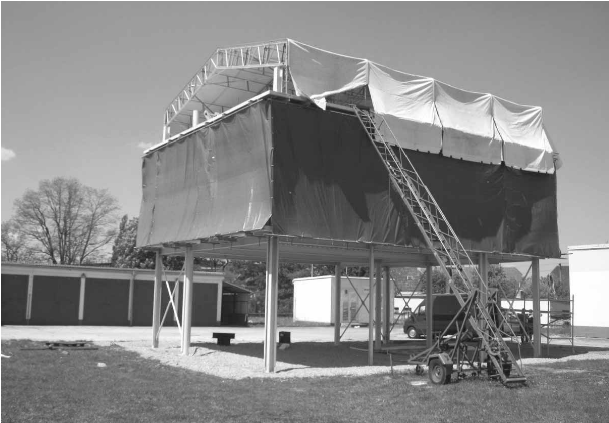
Fig. 29 Temporary covering of the composite slabs
