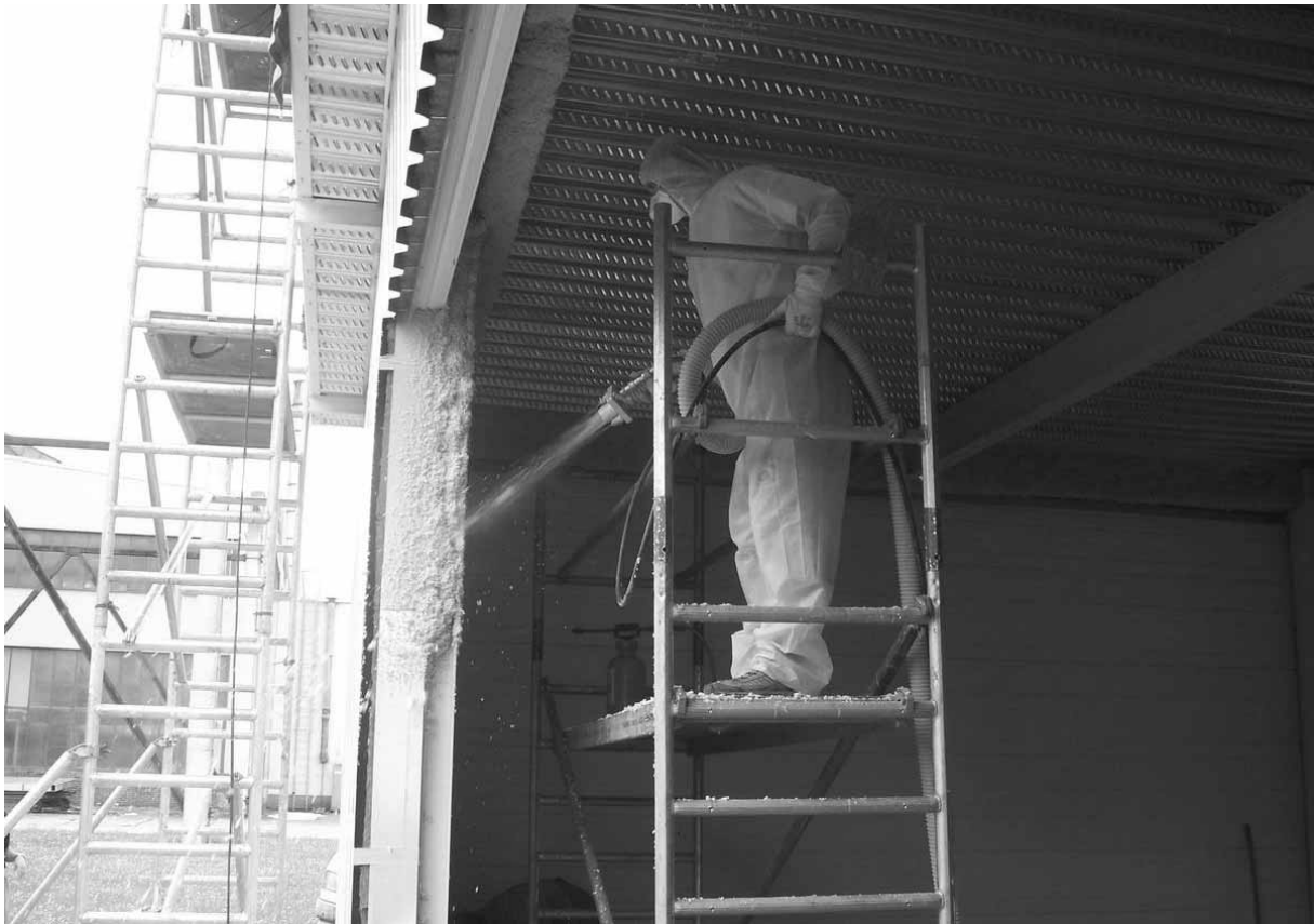
Fig. 31 Application of the fire protection
