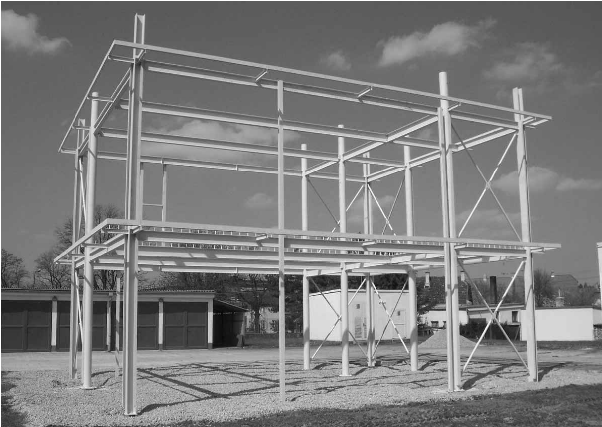
Fig. 26 The complete steel structure
