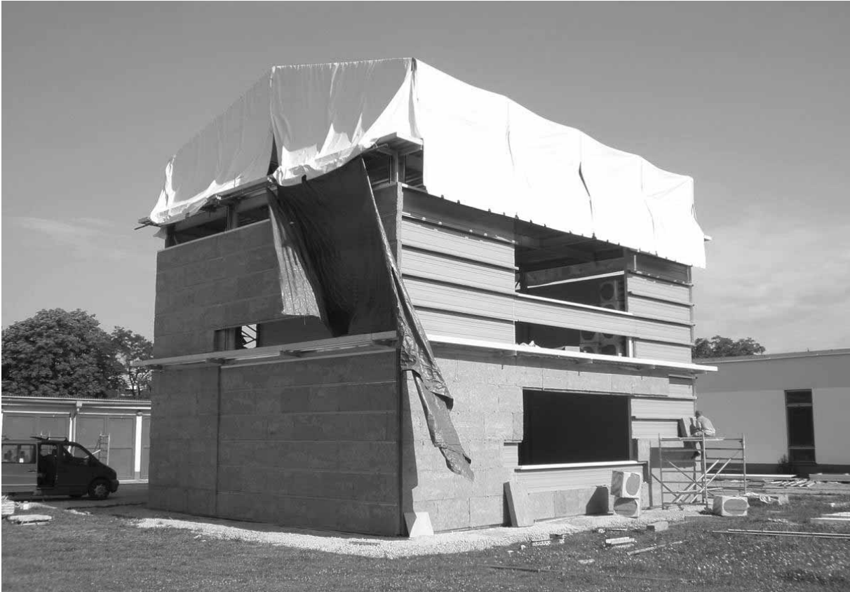
Fig. 30 Installation of the cladding
