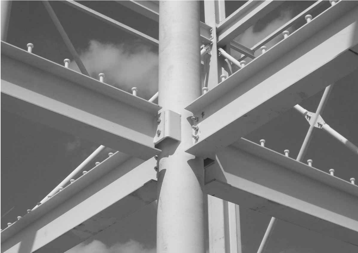
Fig. 27 Reverse channel and fin plate connections
