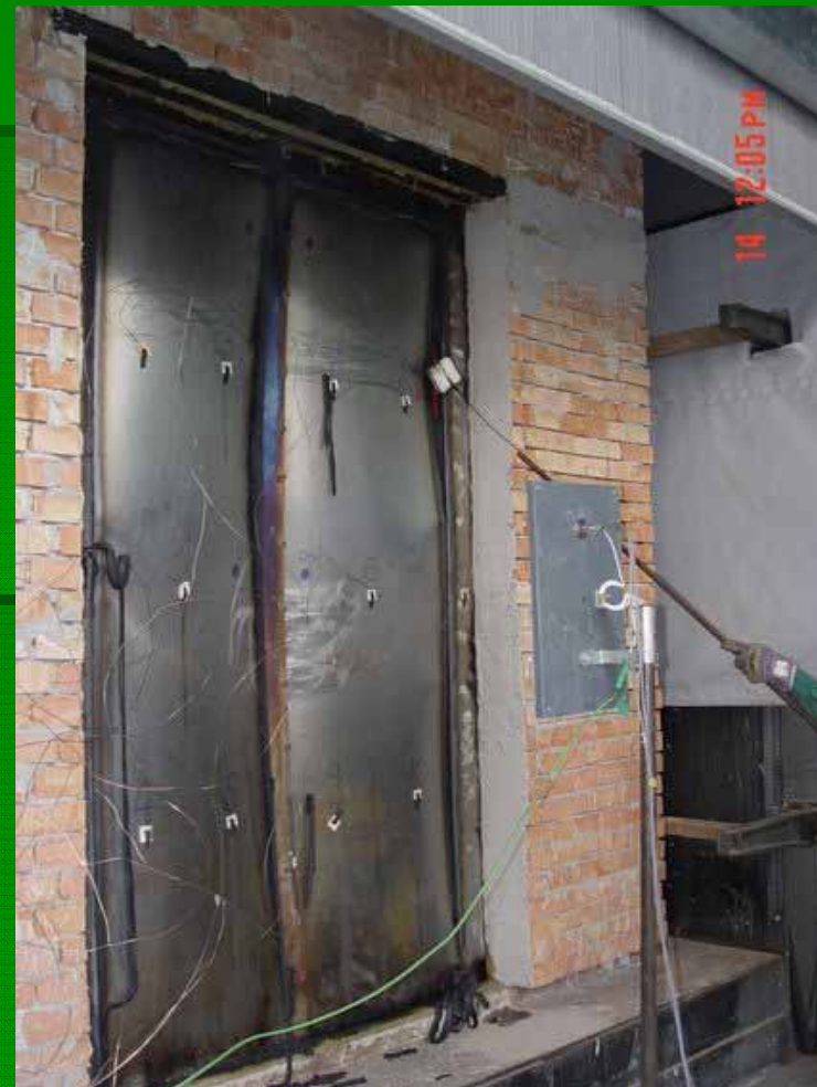
at the end of the fire test
