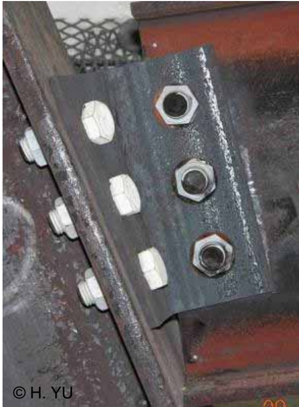
Double web cleat for unprotected beams
