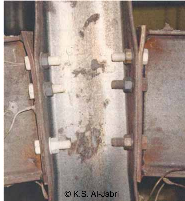
Endplate connections to protected beams framing into columns
