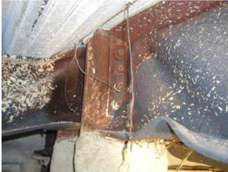
Lower flange buckling occurred during early stages of fire – thermal expansion
