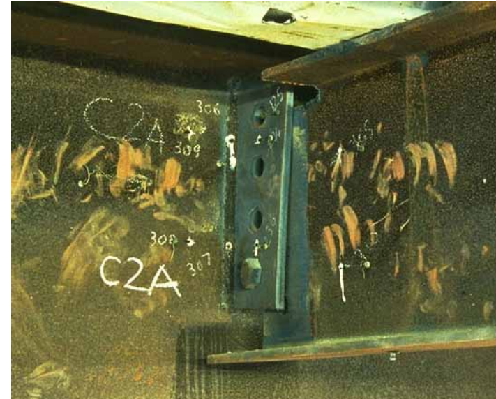
Bolt failure occurred during cooling phase
