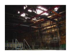
Main structural components of the building have been subjected to high temperatures of varying degrees, depending on the their location in the structural system.
