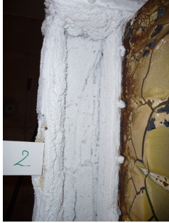
Test specimen no 2 after the fire test.
