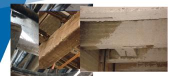
Change of color and structrure of the concrete. Buff color indicate temperaures round 900°C Change of color of the concrete. Red color indicate temperaures round 600°C White color of the surface concrete layers was caused by the chemical reaction between the water, used for extinguishing the fire, and the dehydrated carbonate aggregate
