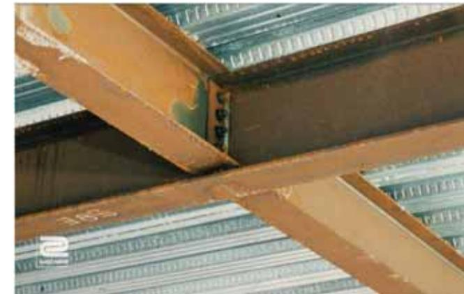
**Beam to beam joint**
