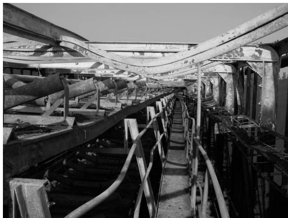
Figure 4.1.5. Deformed upper stiffening truss.
