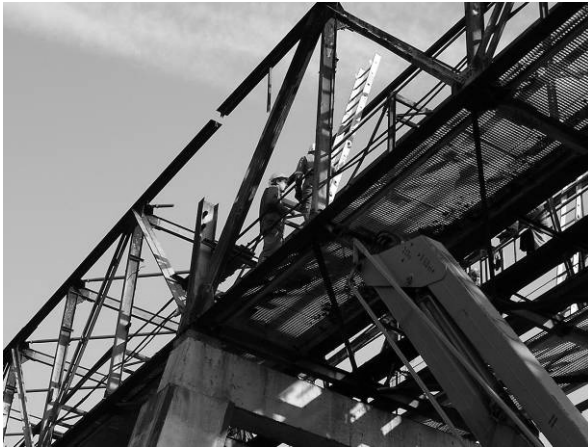
Figure 4.1.7. Replacing of the end frame.
