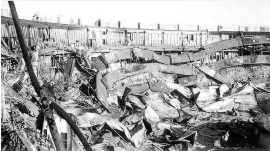
Figure 3.1.4 The structure of the hall after collapse.
