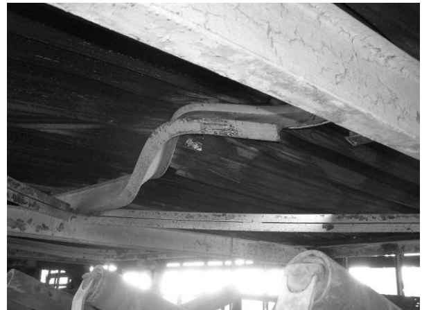
Figure 4.1.6. Deformed purlins.
