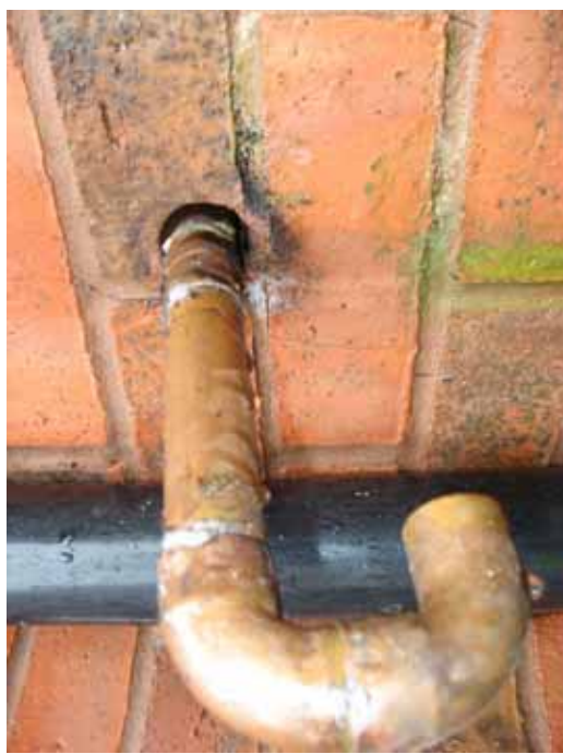
A Timber Framed Building. The fire in the wall cavity destroyed the building. Caused by brazing a copper pipe
