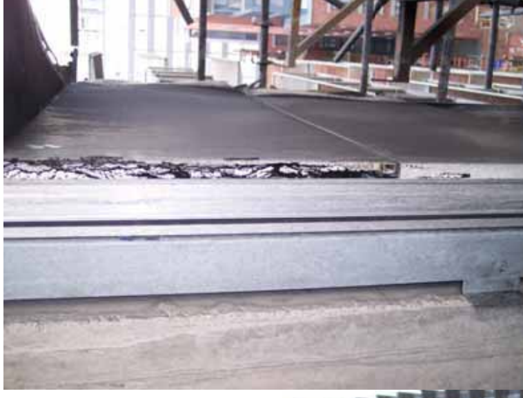
The Edge, Salford. Fire spread up the outside of the building in 30 seconds due to flammable cladding
