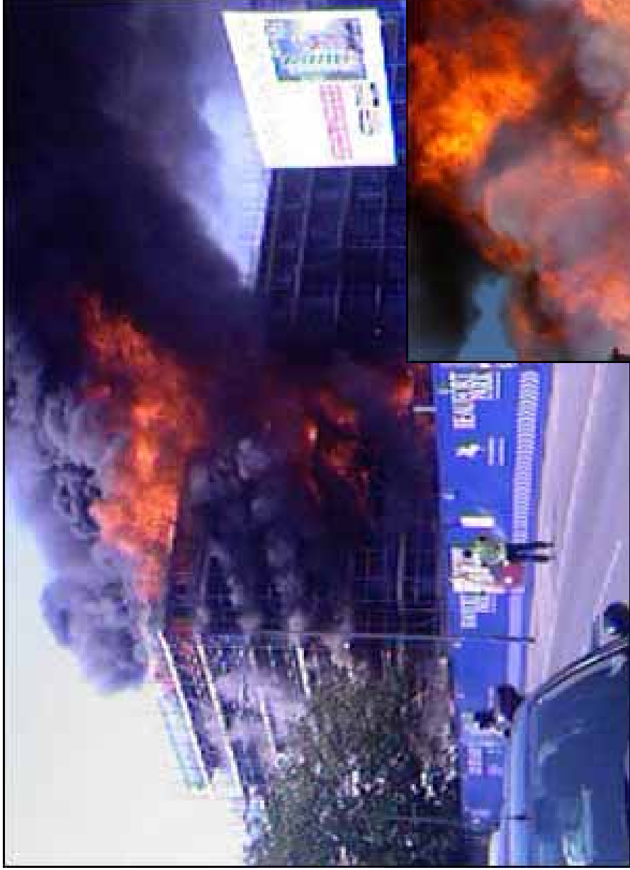
Collingdale Fire, London. Timber Framed Building under Construction. Took just a few minutes to burn to the ground
