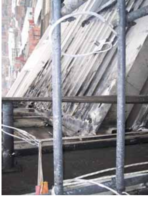
The Edge, Salford. Fire spread up the outside of the building in 30 seconds due to flammable cladding
