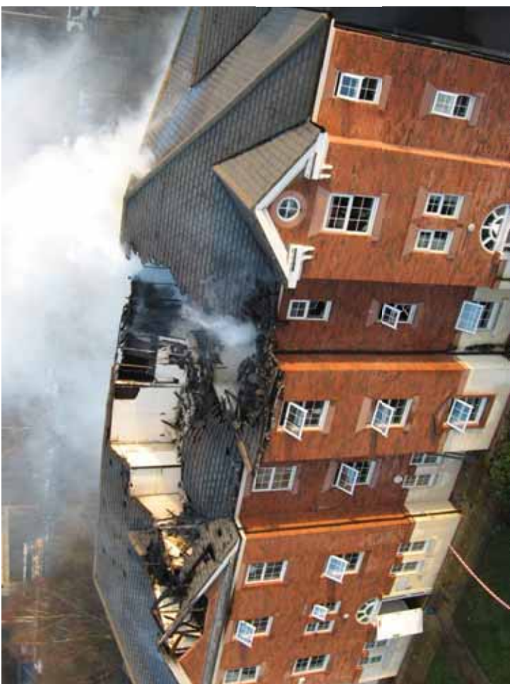
A Timber Framed Building. The fire in the wall cavity destroyed the building. Caused by brazing a copper pipe
