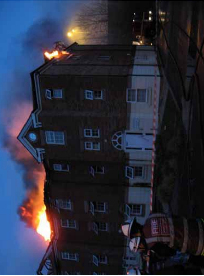
A Timber Framed Building. The fire in the wall cavity destroyed the building. Caused by brazing a copper pipe
