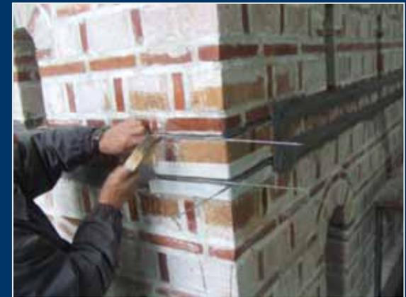
the grooved part of the joint was filled with epoxy resin
