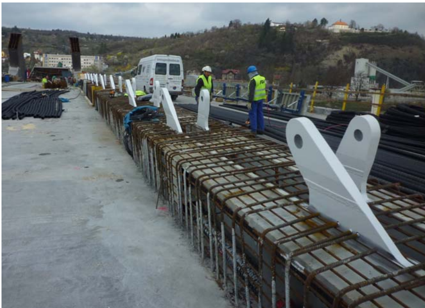
Fig. 8. Deck chords before concrete casting
