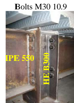
Fig. 3. Composite beam-to-column joint
