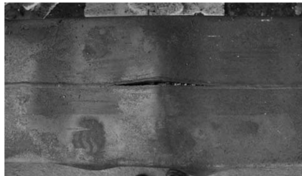
Fig. 2 Fracture of the weld in a concrete filled steel tubular column fire test
