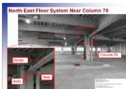
Figure 2: Seated connection to column 79 in WTC7 (FEMA 2008)
