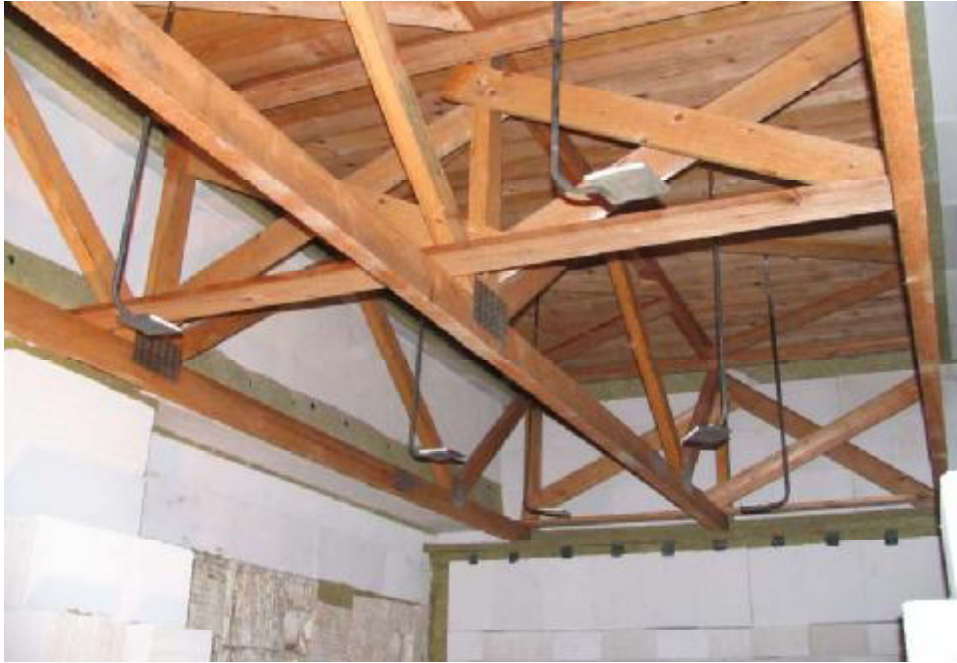
Fig.2. Structure No. 1 before the fire test
