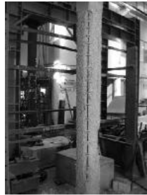
Fig. 10. Column C4 after test
