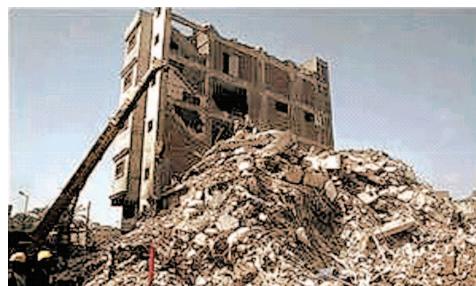
6-Story Reinforced Concrete Textile Factory in Alexandria, Egypt, July 19, 2000
