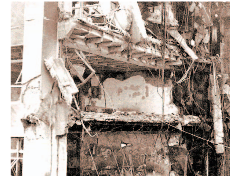
21-Story Reinforced Concrete Office Building, in Sao Paulo, Brazil May 21, 1987
