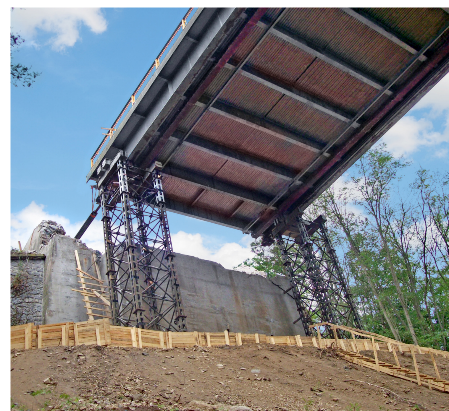
Demolished upper part of the abutment
