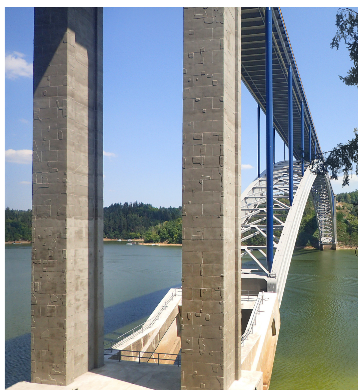
Žďákov Bridge, view on the arch
