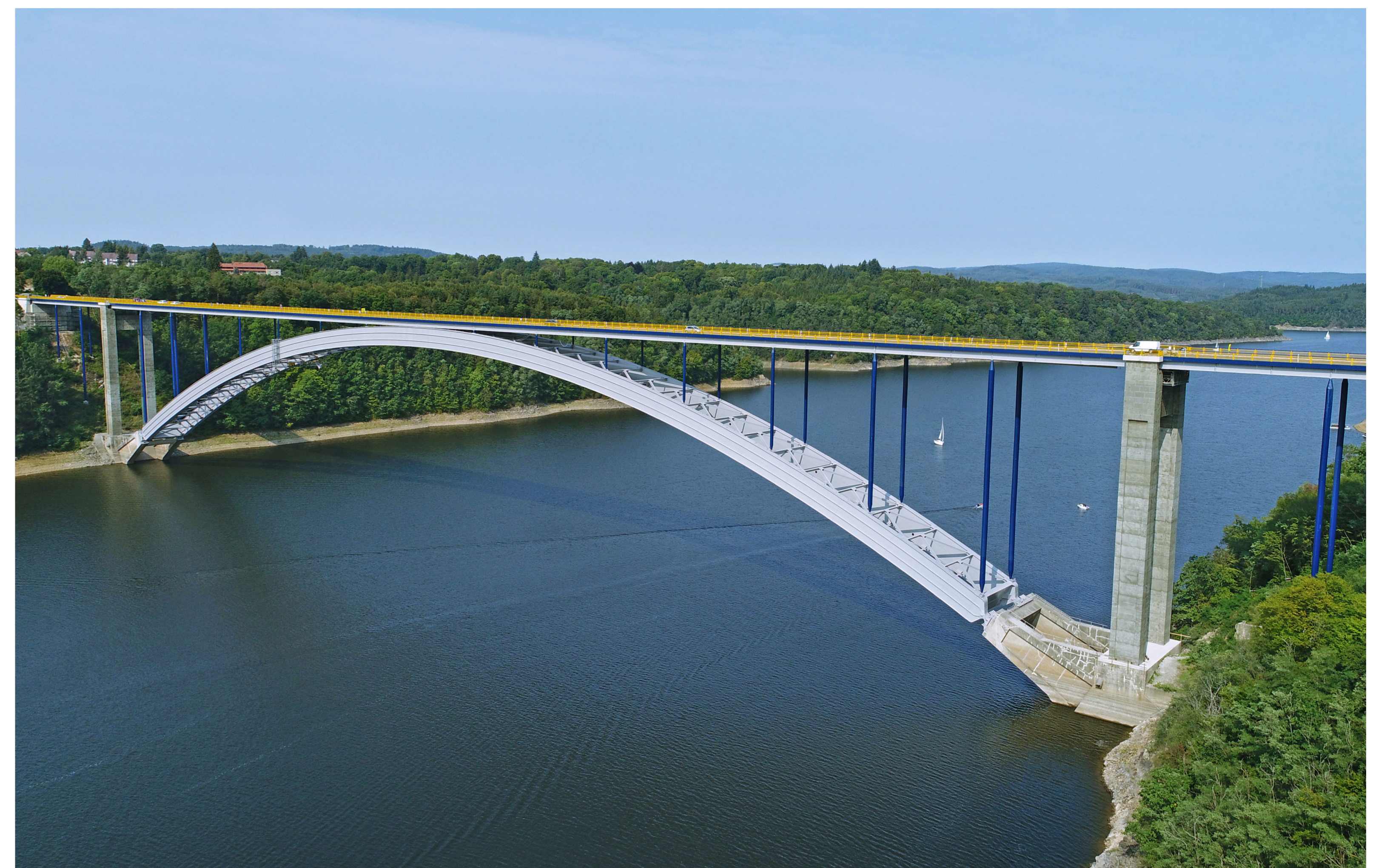
Žďákov Bridge over the Vltava River from 1967
