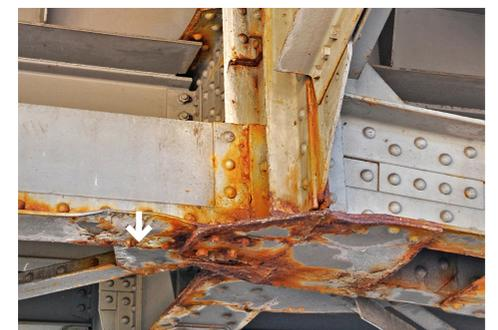
Corrosion of members in the detail of the embedded hinge, excessive def
