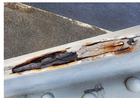
Diagonal deformation due to crevice corrosion
