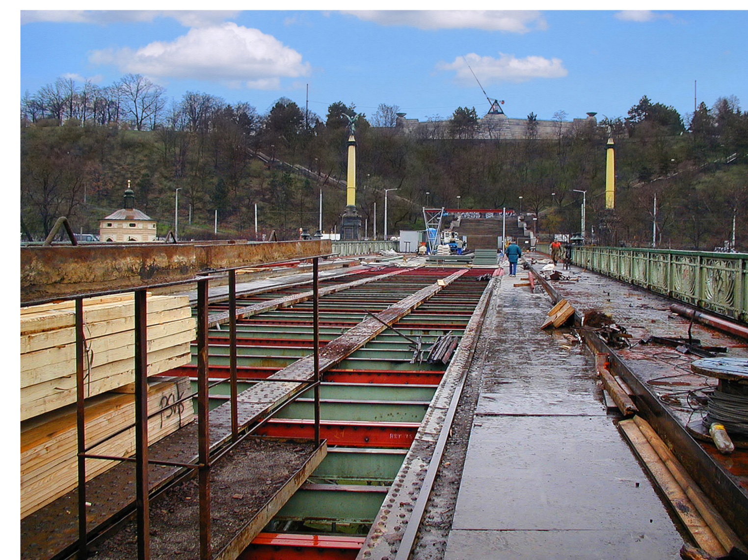
View of the bridge deck during reconstruction in 2000–2001
