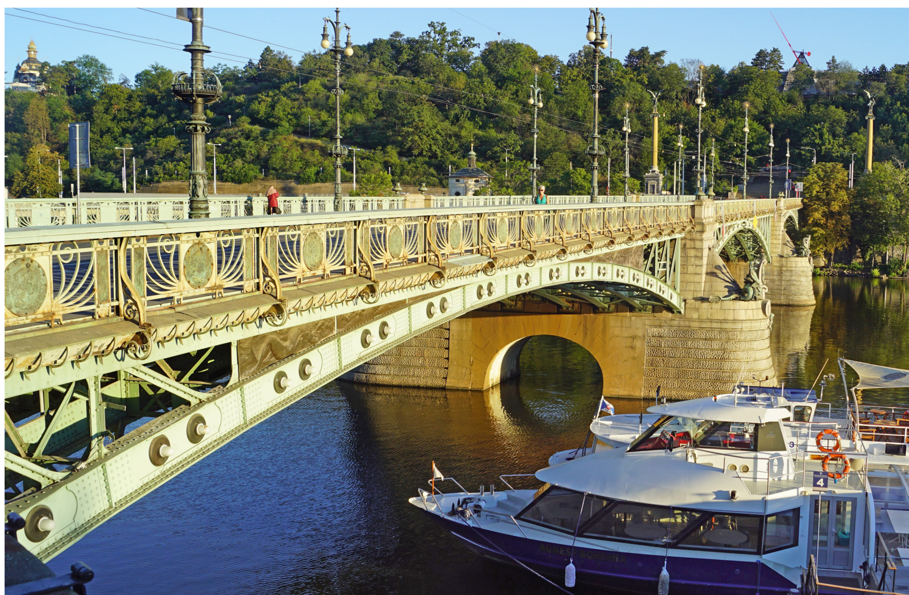
View of the bridge from the west in 2020
