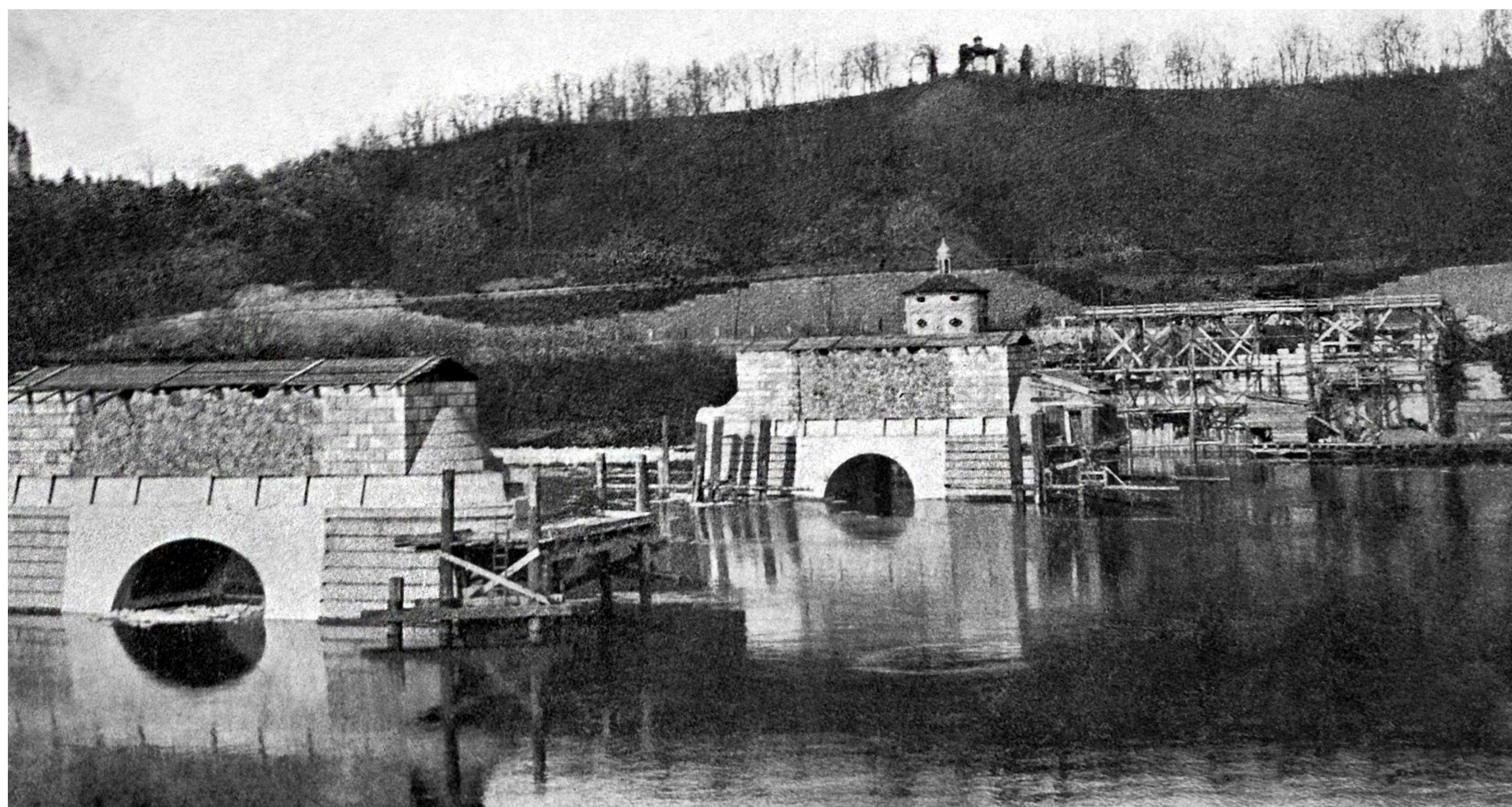
The bridge substructure construction
