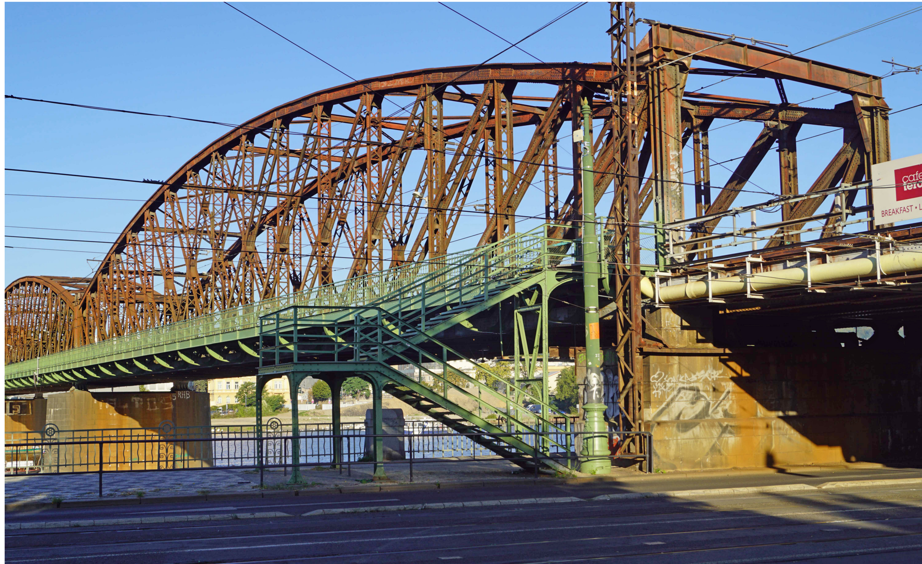
View of the bridge from the southeast in 2021
