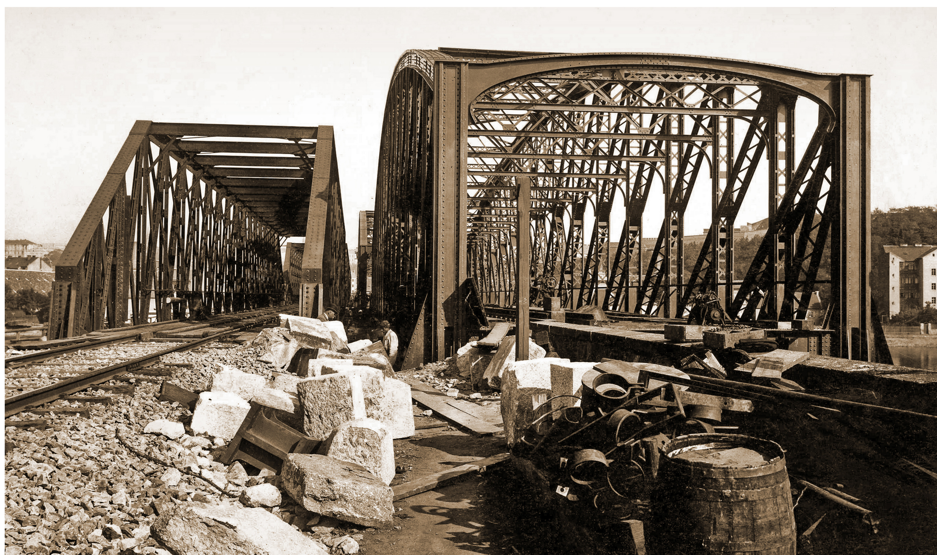
Replacement of bridge in 1901
