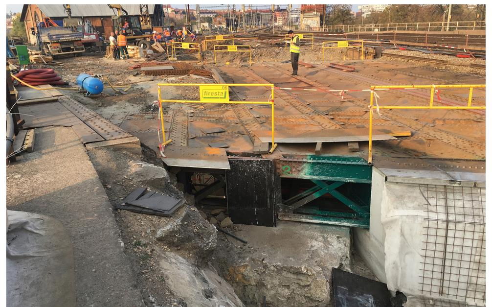
The bridge deck and coating of the end cross beam
